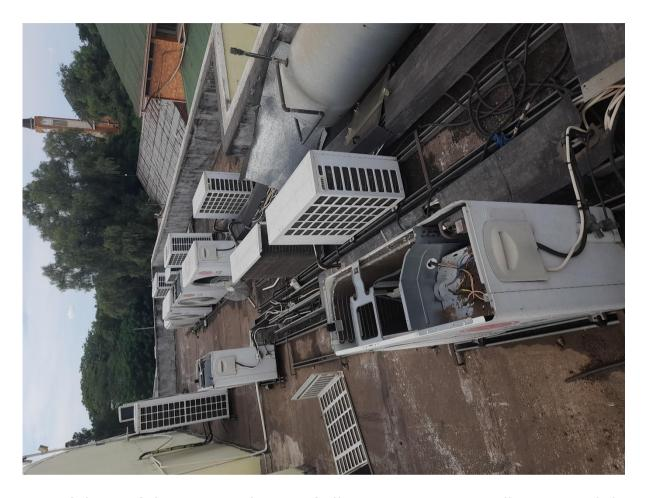
Top of the roof the Municipality, roof all Air cons are not well connected they need to be re wired.
