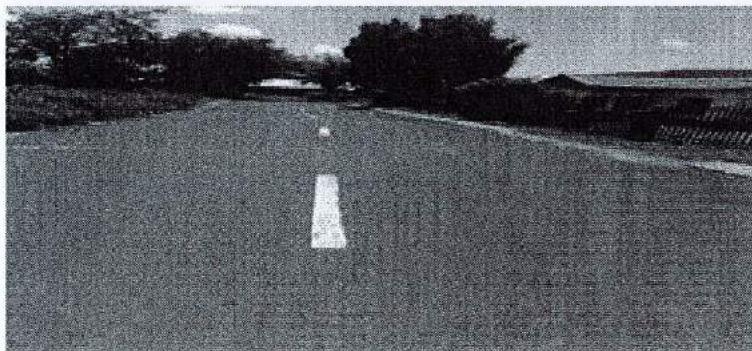
Figure 7: Dinokana Ward 10 Internal Road
